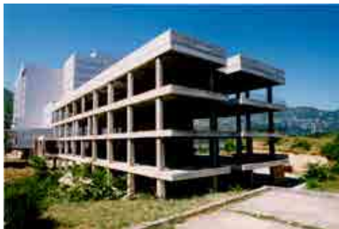
IZGRADNJA ZGRADE MEDICINSKOG FAKULTATA CONSTRUCTION OF THE BUILDING OF THE SCHOOL OF MEDICINE
